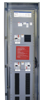
Wall-mount maintenance bypass panel
