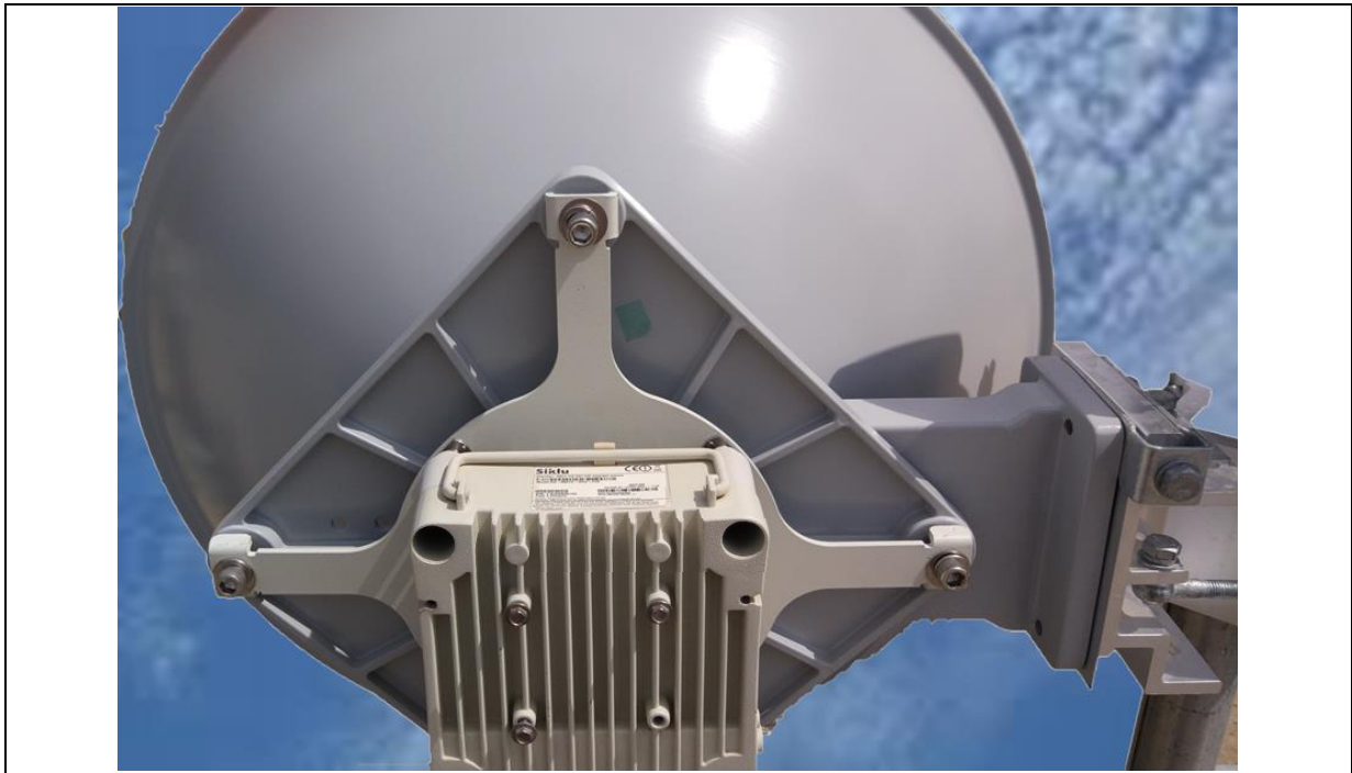
FIGURE 3a: 2FT Antenna installation (EH-ANT-2ft60GHz)
