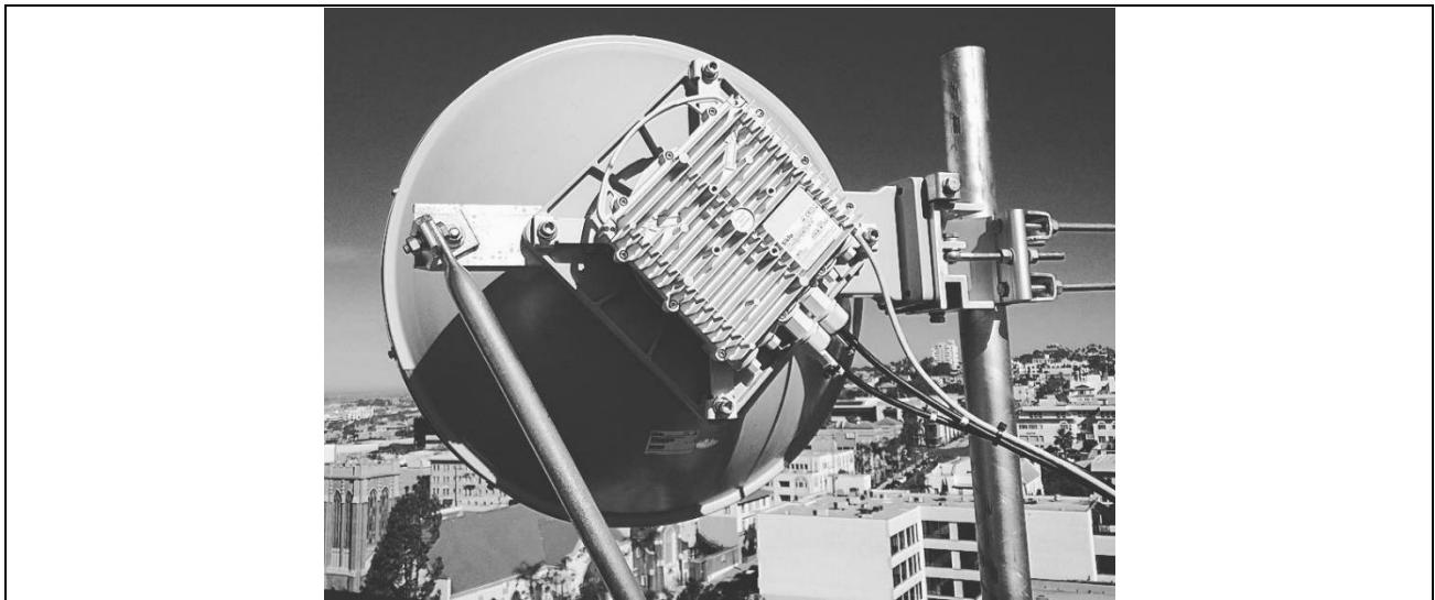
FIGURE 2a: Typical installation (without 5GHz radio or Siklu mount)
