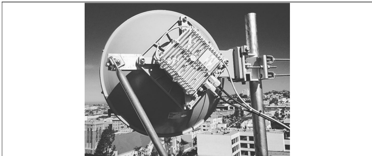
FIGURE 4a: 2FT Antenna installation (EH-ANT-2ft-B)
