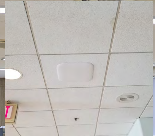
Oberon Envelop™ Model 1040 recess mount for suspended and cloud ceilings conceals the AP behind a low-loss, low-profile plastic cover
